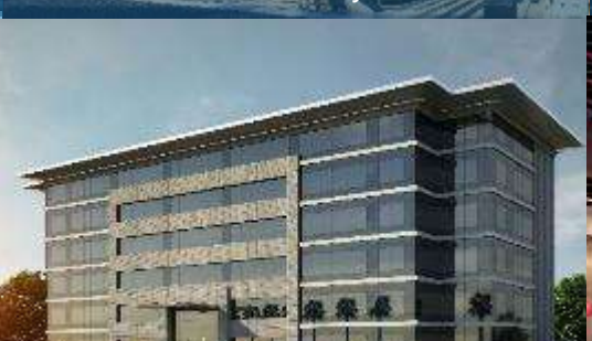
South-West Office Building – CFC
