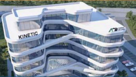
Kinetic Office Building, Smart Village
