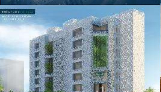
EG Bank Headquarters, New Cairo
